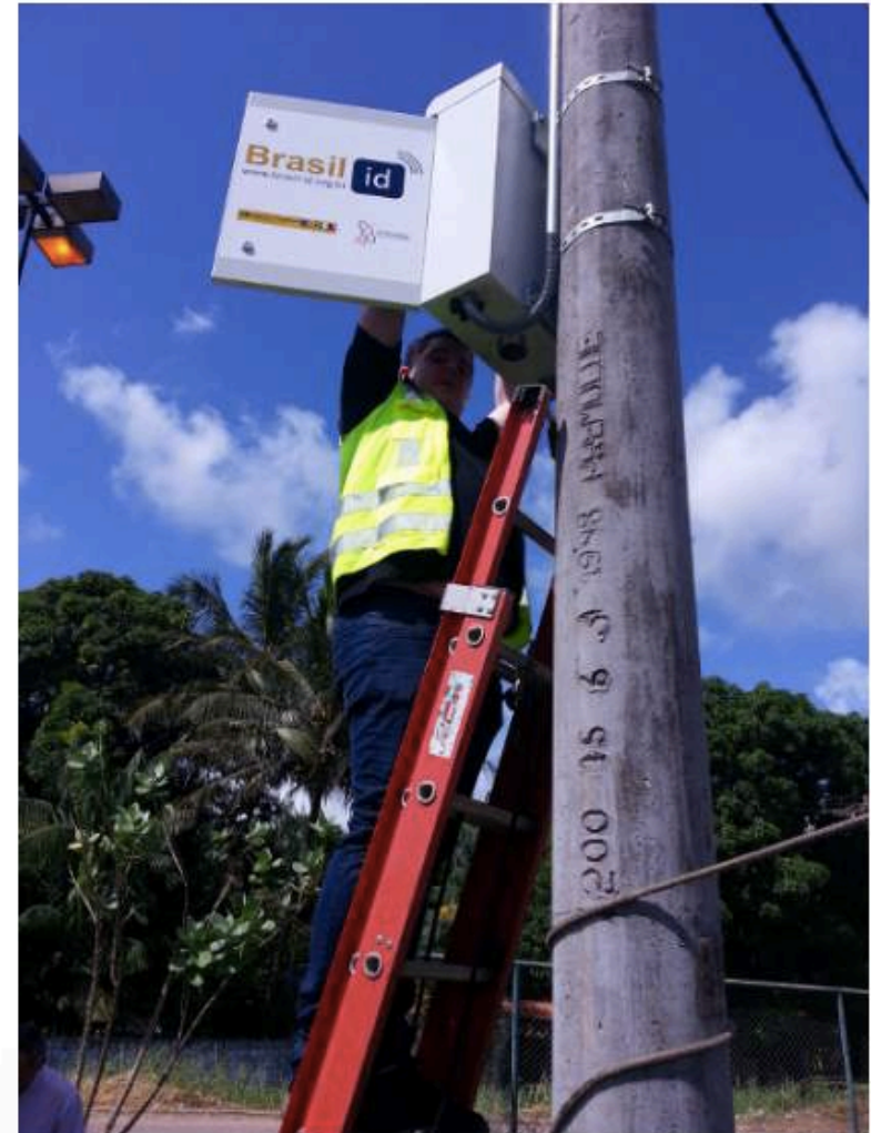
Tag Initialization Equipment for Field Operations and a Brasil-ID Reading/Writing Systems which is connected to the Central BackOffice for security and Access Keys management
